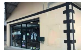
Renforcement parasismique
